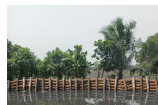
Coir based embankment reinforcements to address flooding issues using local expertise
