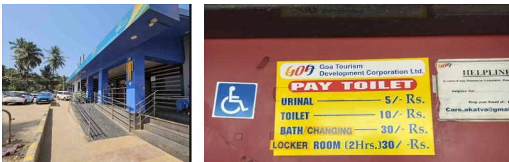
Photo of an Aspirational Public Toilet near Palolem Beach
