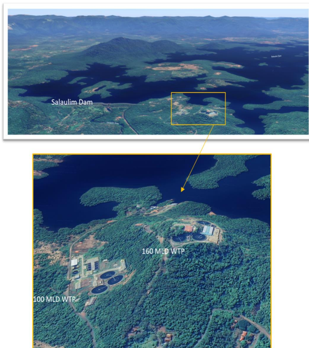
Figure 19: Location of Salaulim dam and Water treatment plant on a hillock.
