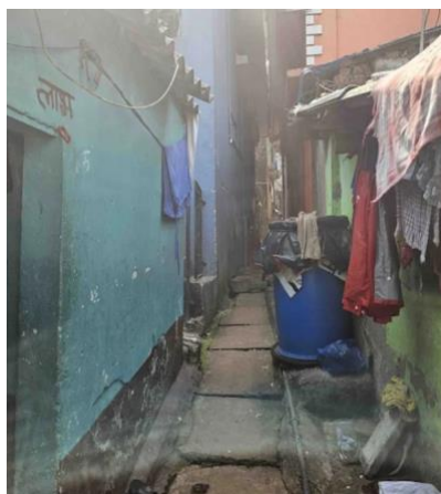
Sewerage connection lines to the households
