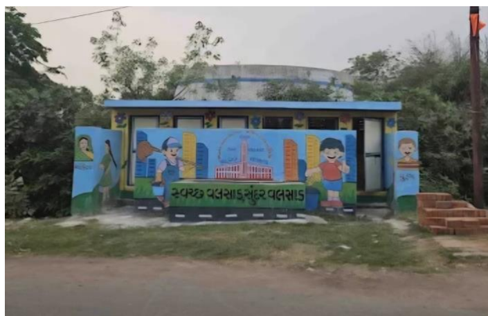
Photo 1 : Community toilet in Valsad City
