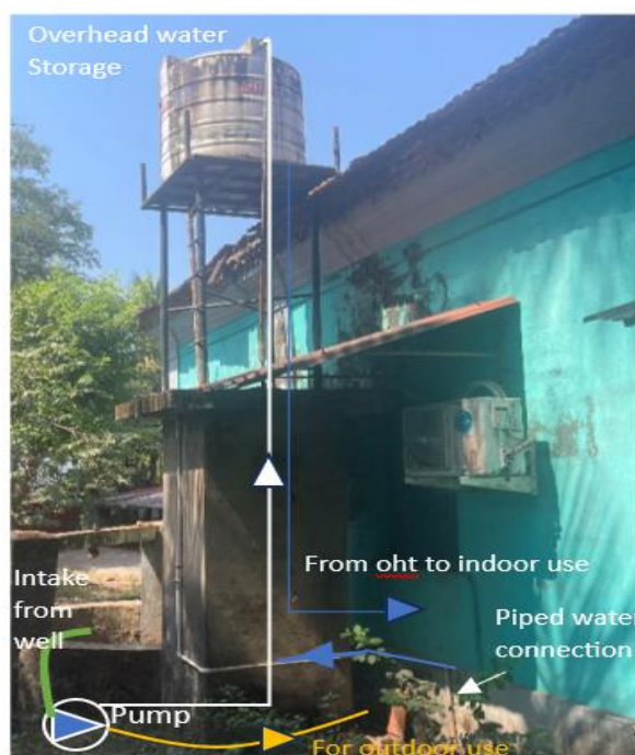
Figure 12: Water-supply Infrastructure at household
