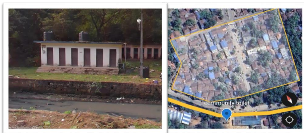
Photo: Community Toilet in Low-income Locality
